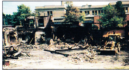
A demolition crew clears the charred remains of Keasling's Drug Store.
